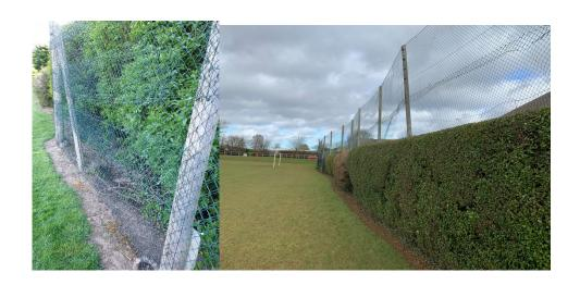
The Ball Stop fence at St David's (thought to be around 8 metres high) is deteriorating. The wire mesh netting is no longer effective and some of the telegraph poles are in need of replacement. (One snapped at the base recently) The fence is approximately 90 metres long.
